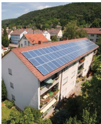
Photovoltaik-Anlage in Rohrbach
